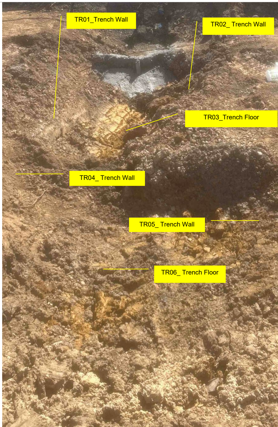
Pipe Trench excavation
